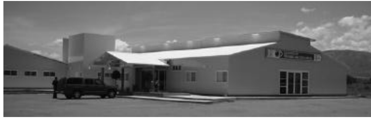
Exterior and interior views of Guanajuato's brand new Centro de Rehabilitacion.
